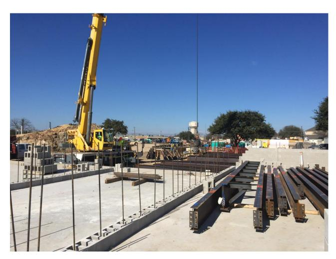
STRUCTURAL – Structural columns and beams are being positioned for erection at the Athletic areas.
