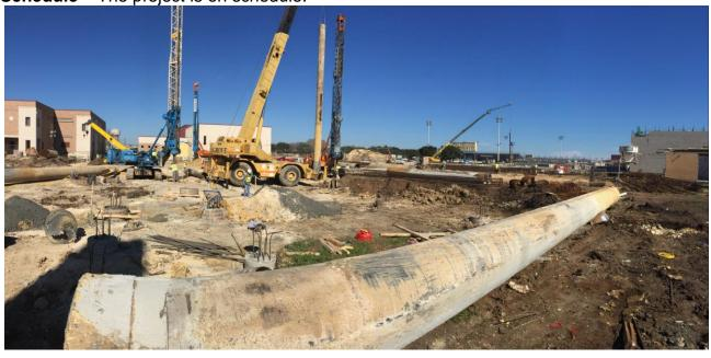
**FOUNDATION & PIERS** – Pier drilling continues between the current high school Administration Building and the Band Hall. Steel casing is being used during the pier concrete pours due to the presence of ground water.
